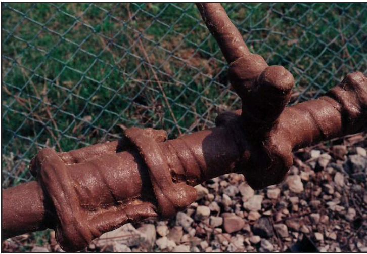
#1 Wax-Tape applied to coupling, street tee and leak clamp.
