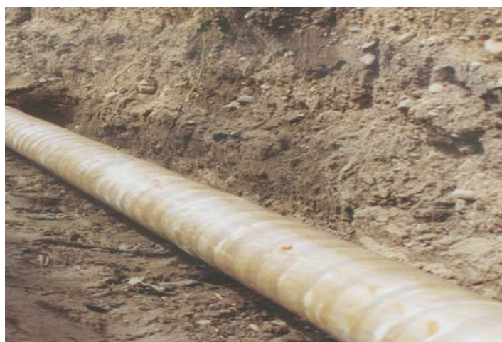
Section of 16" pipe reconditioned using #1 Wax-Tape.
