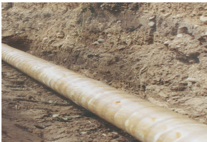
Section of 16" pipe reconditioned using #1 Wax-Tape.
